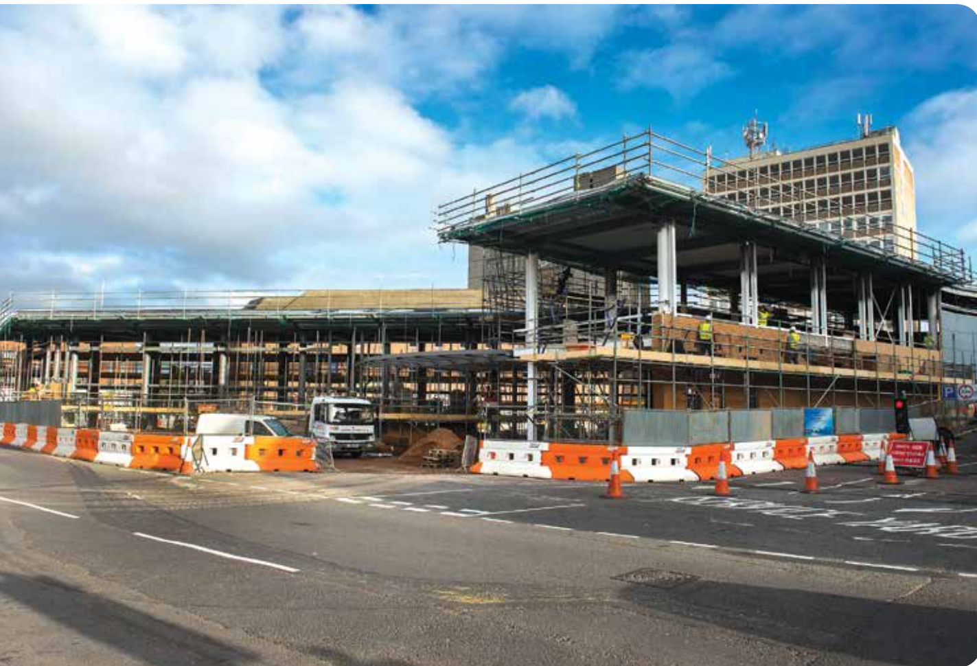
The new Haymarket Bus Station being constructed
