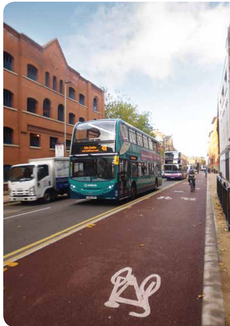
Example of new cycling infrastructure improvements.
