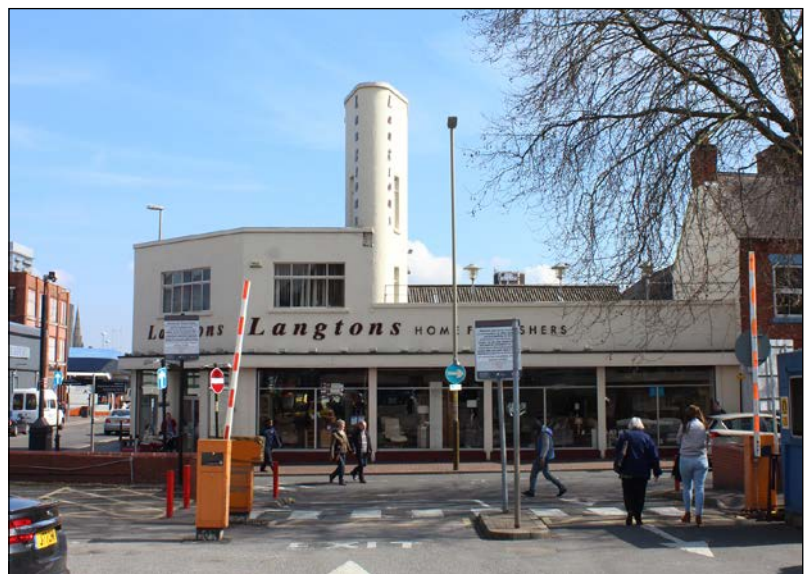
81 Church Gate is one of two former car garages in the area, the distinctive ‘fin’ forms an interesting corner feature
