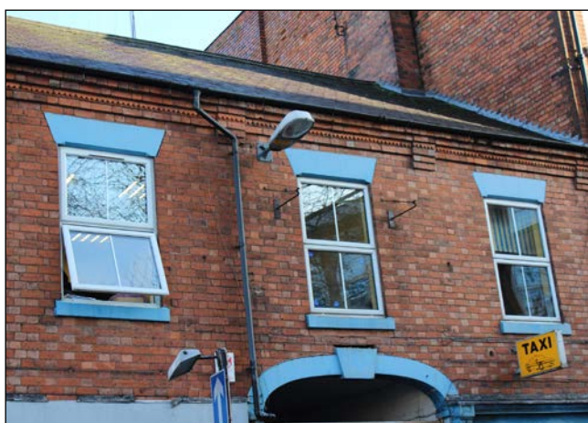
Inappropriate windows at 79 Church Gate.
