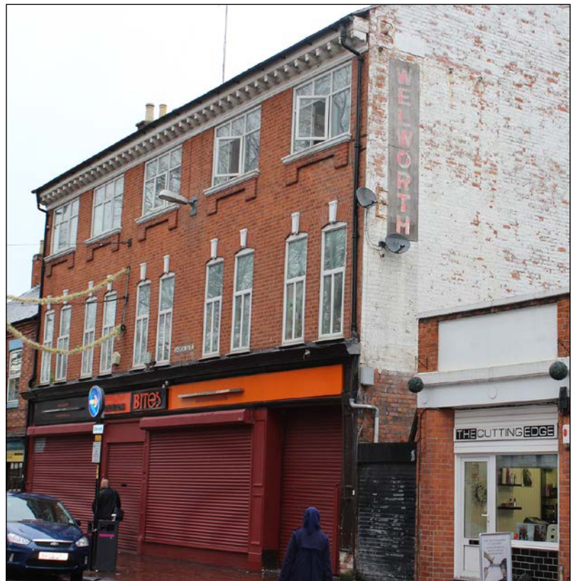
Former coach workshop at 75 Church Gate.
