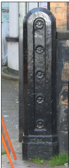
Cast Iron gate pier at 66 Church Gate.
