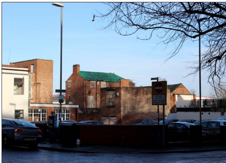
The car part at the corner of Butt Close Lane and East Bond Street suffers from a lack of activity and poor landscaping.
