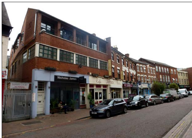
7 East Bond Street is a former vehicle garage which has been extended and converted to shops and flats.
