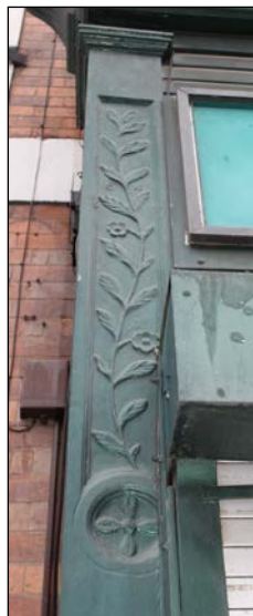
Iron Pilaster at 62 Church Gate.
