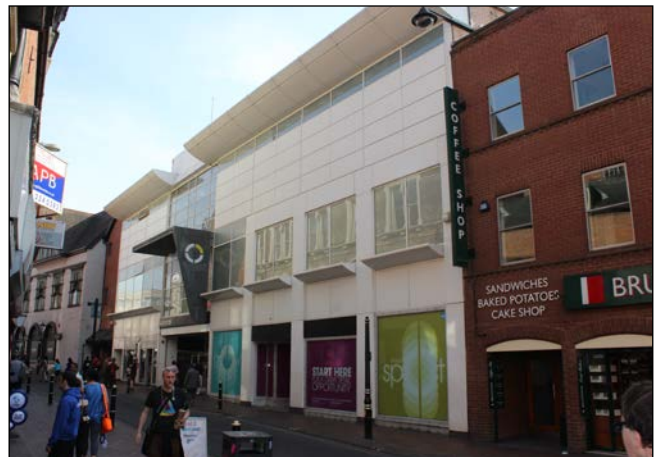
Flat and uninspiring façade to Highcross on Church Gate.
