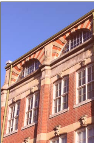
Brick and stonework on 13-21 Church Gate.
