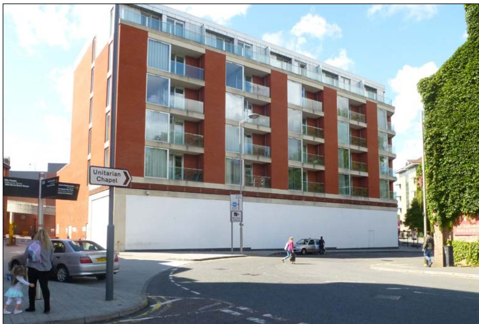
Flats on East Bond Street, which form part of the Highcross forms a strong edge to the conservation area although is not being within the boundary. The buildings was constructed over the former route of St Peters Lane.
