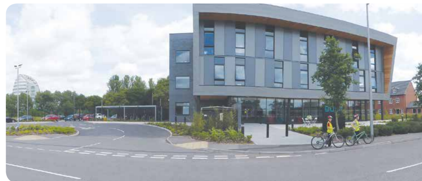
The city council's new Dock building with landscaping to manage drainage
