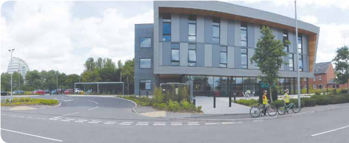
The city council's new Dock building with landscaping to manage drainage
