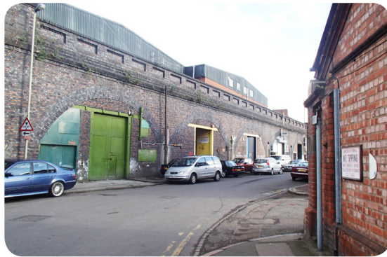
Viaduct arches on Jarvis Street
