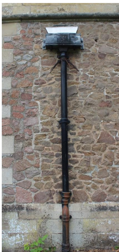
Left: The cast iron downpipe with a stamped rainwater hopper at St Peter's Church.
