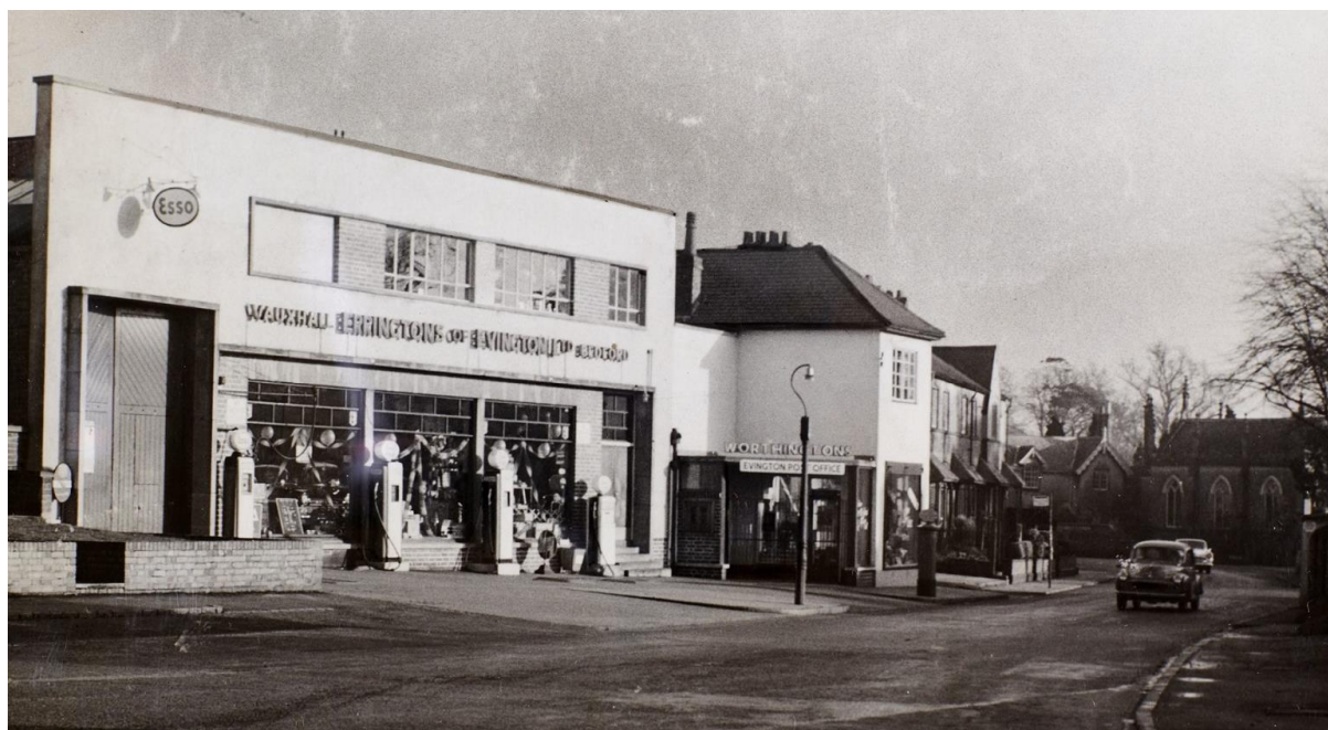
The same view circa 1955, the cottages have been replaced by a vehicular garage and petrol pumps. The garage would be redeveloped for the current flats in the early 00's.
