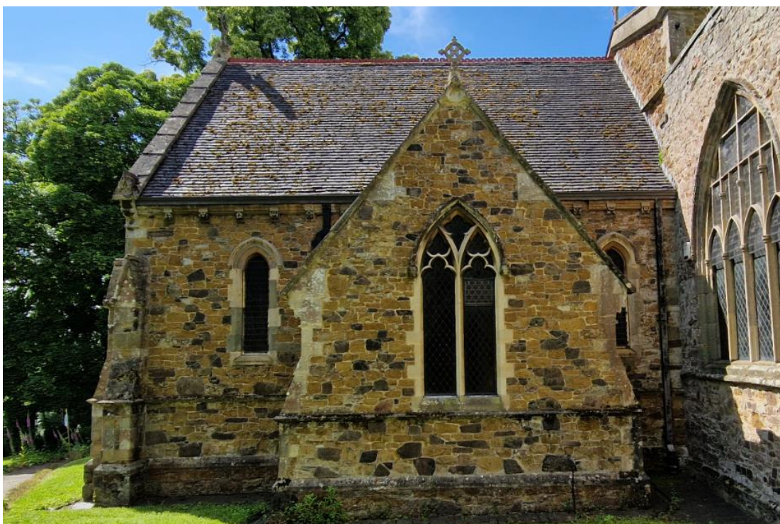
The Church of St Denys contains a variation of local building stones.
