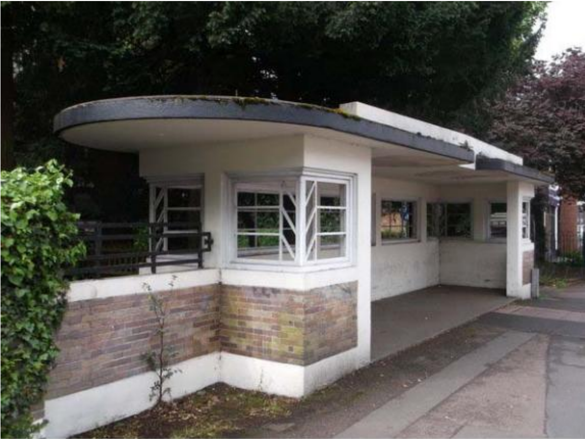
Figure 31: Tram Shelter to the West of Humberstone Park
