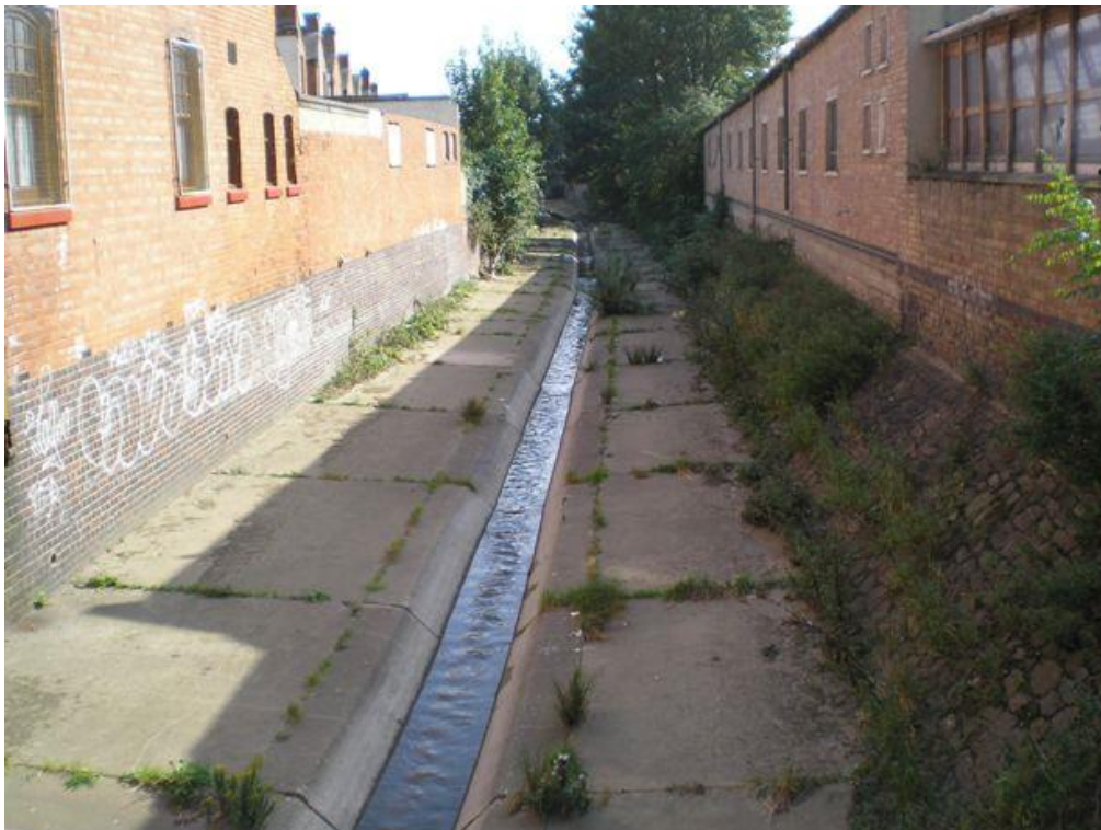
Figure 25: Example of Concrete Channels along Willow Brook
