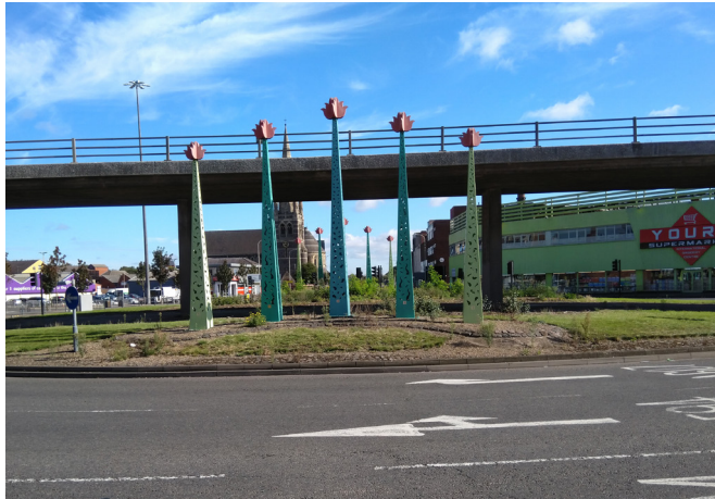
1. Existing image of Burleys Way roundabout and underpass.
