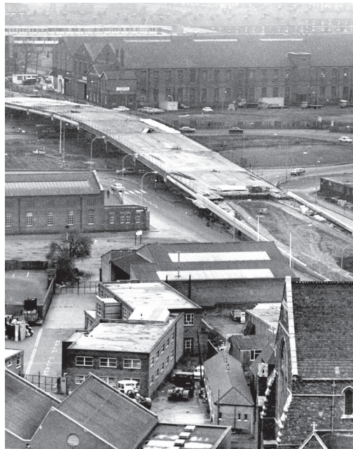
Construction of Belgrave Road flyover 1973 (Leicester Mercury)
