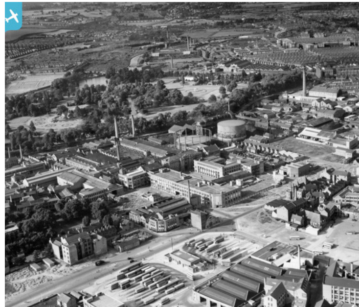
Leicester viewed from the air in 1947 showing St. Margaret's Bus Station and the associated garages. (Historic England)
