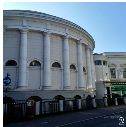
2. Belvoir Street Chapel
