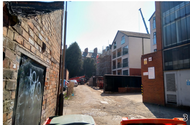
3. The rear of the block north of the Oval.
