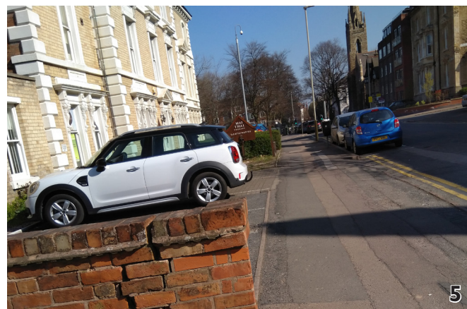
5. Example of boundary removal for parking on University Road.
