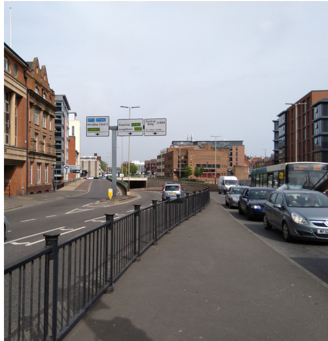
1. Ring Road, Southgates Underpass
