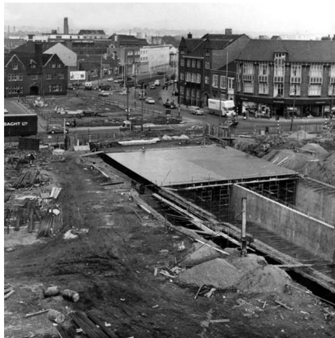
Construction of the underpass in the 1960s. As can be seen many of the blocks adjacent to Southgates had been cleared. (Leicester Mercury)
