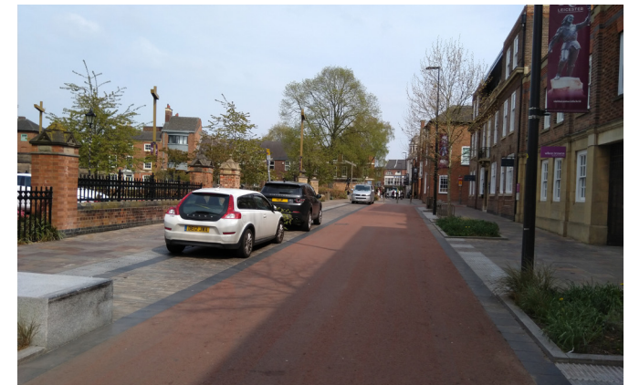
4. St. Martins/Peacock Lane after Connecting Leicester improvements
