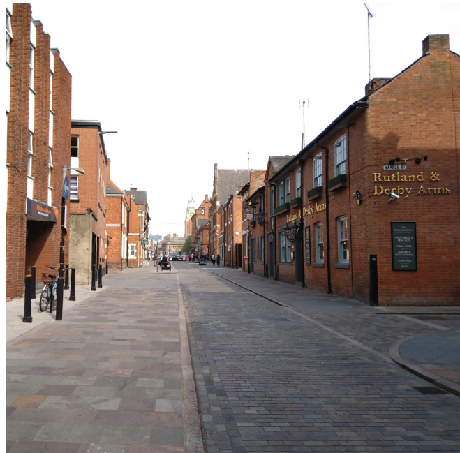
3. Centre Calmed Street, Millstone Lane
