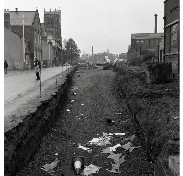
Construction of St. Margaret's Way 1969 (Leicester City Council)
