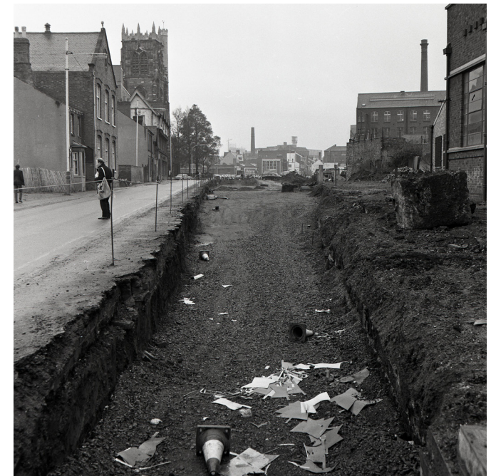
Construction of St. Margaret's Way, 1969
