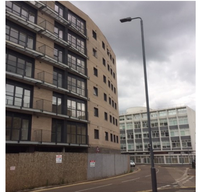
Leicester House (A) currently under construction at 7 storeys.
