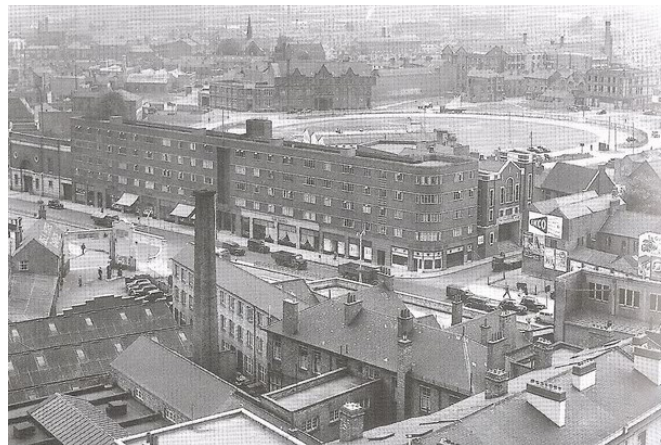
View of Charles Street and the Lee Circle surface car park (Leicester City Council)
