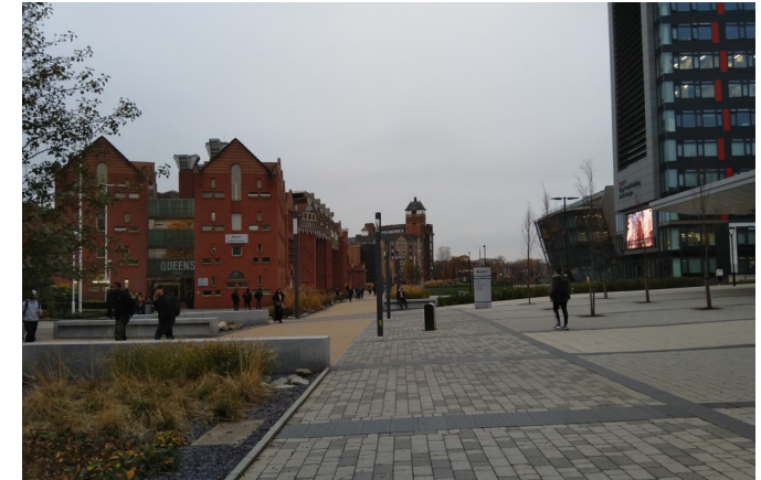
3. Mill Lane, DMU following Connecting Leicester Improvements 2019
