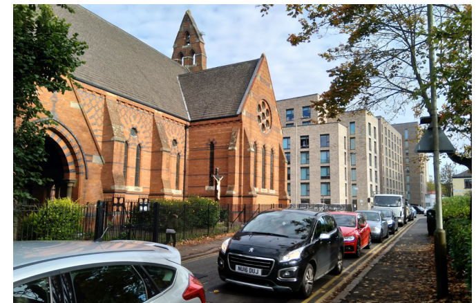
4. View of the Church's frontage when looking east along Jarrom Street.
