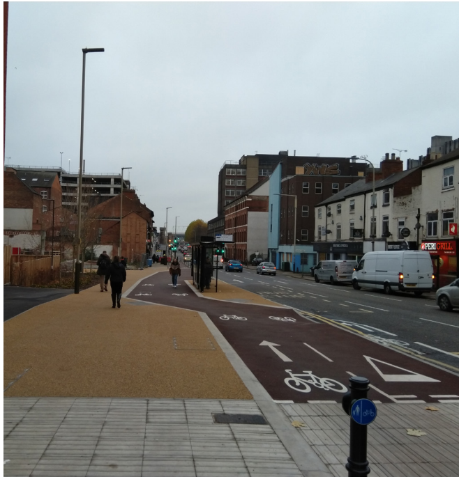
1. Centre Connector Hub, Welford Road
