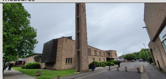
Figure 3: Community facility within the centre
