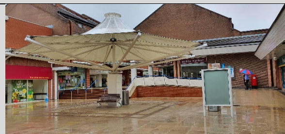
Figure 2: External Pedestrian Walkway
