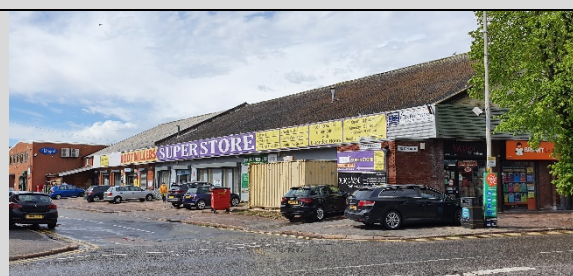
Figure 3: Melton Road Discount Store
