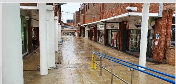
Figure 3: External Pedestrian Walkway
