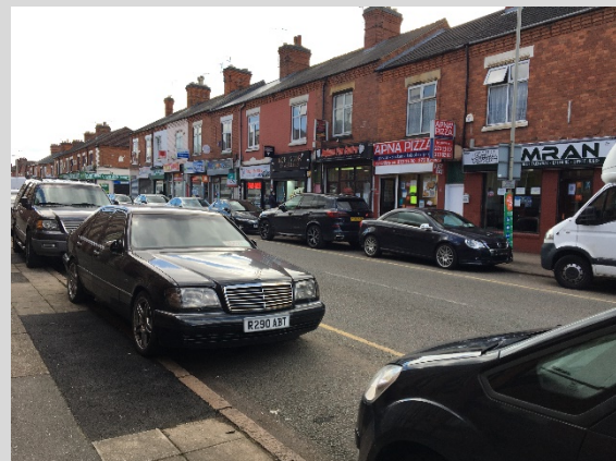
Figure 2: Saint Saviours Road (West) is a linear centre, consisting largely of converted former terraced properties. As such, car parking within the centre is of limited availability
