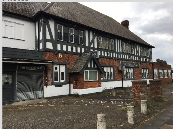
Figure 1: The Duncan Road Social Club/Saffron Lane Estate Working Men's Club & Institute has limited activity during the day
