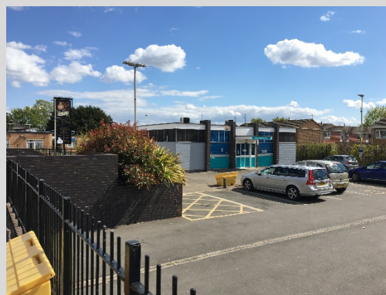
Figure 2: Rushey Mead Library (and the adjacent Rushey Mead Health Centre) provide a strong element of community uses at the local centre
