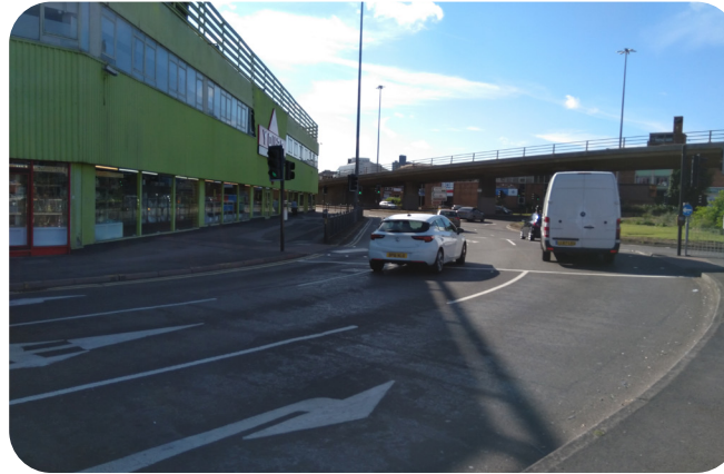
Figure 39: Ring Road, Burleys Way/ St Matthews Way
