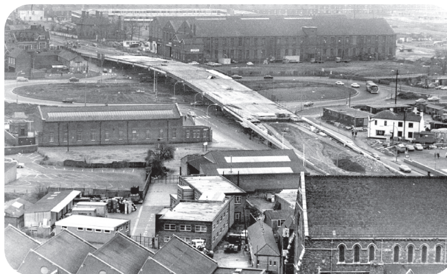
Figure 22: Construction of Belgrave Road Flyover 1973 (Leicester Mercury)
