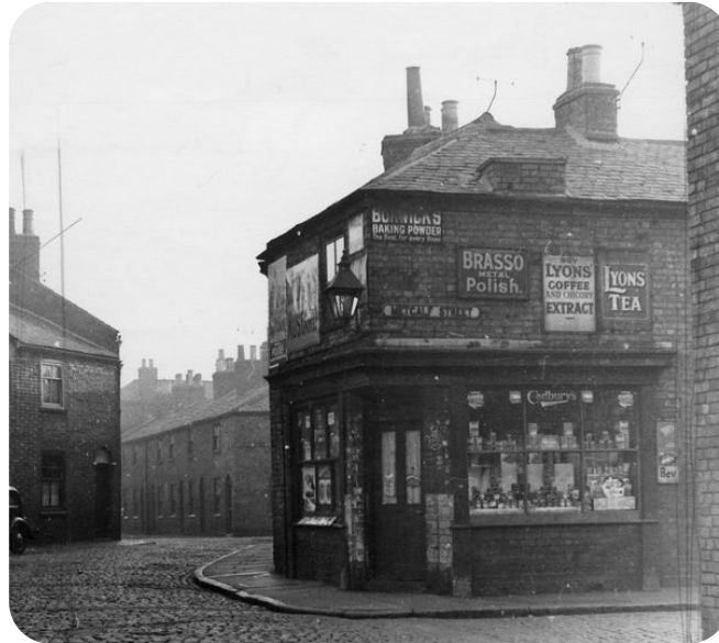
Figure 15: The junction of Metcalf Street & Lead Street, Leicester. Lead Street's junction with Carley Street is in the distance, pre 1950s. These streets no longer exist (Leicester Mercury)
