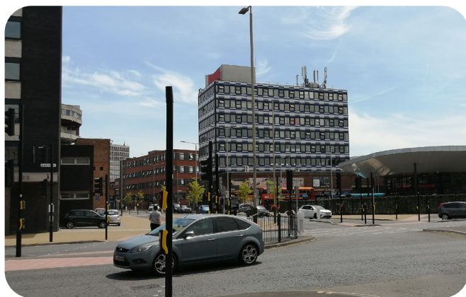
Figure 33: Corner of Abbey & Gravel Street
