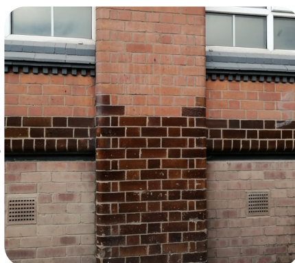
Glazed Brick Plinths
