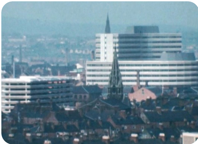
Figure 13: New Walk Centre Newly Built, Image from 1975 (ITV News Central)
