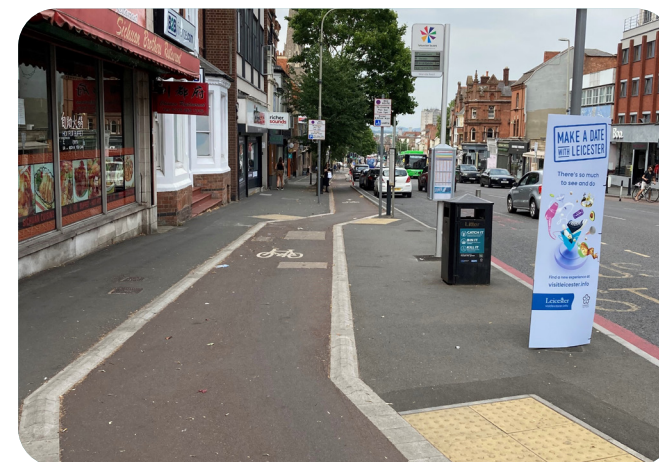
Figure 59: London Road after Connecting Leicester Improvements
