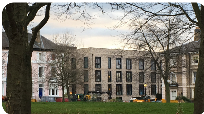
Figure 25: 67-75 Princess Road East (20160758) - from New Walk Promenade Across De Montfort Square.
