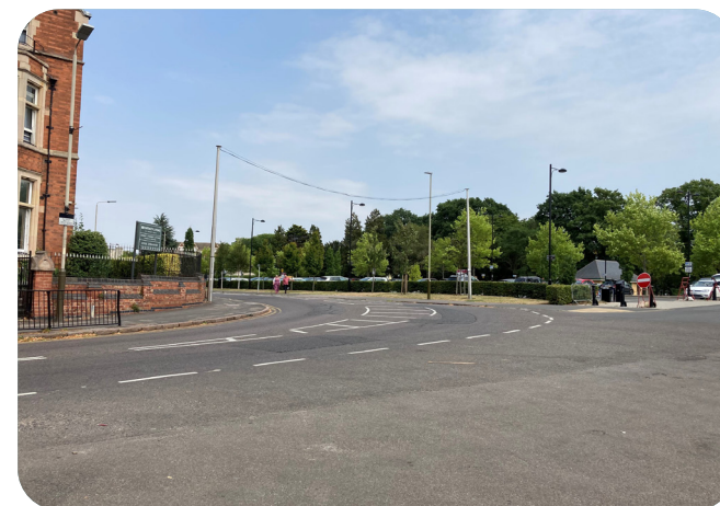
Figure 54: Junction of Granville Road and Regent Road .....
