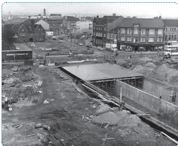
Figure 9: Underpass Construction in the 1960s - Many of the Adjacent to Southgates Blocks had been cleared. (Leicester Mercury)
