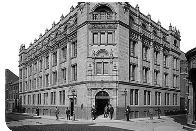
Figure 16: Faire Brothers & Co. Bootlace Warehouse on the Corner of Rutland Street & Southampton Street 1901 (Historic England Image Archive).
