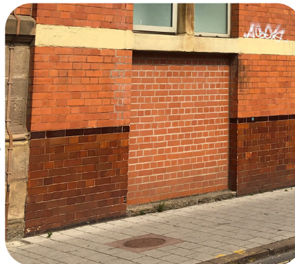
Glazed Brick Plinths
