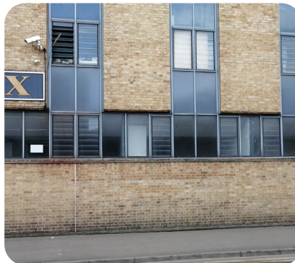
Framing of Windows
