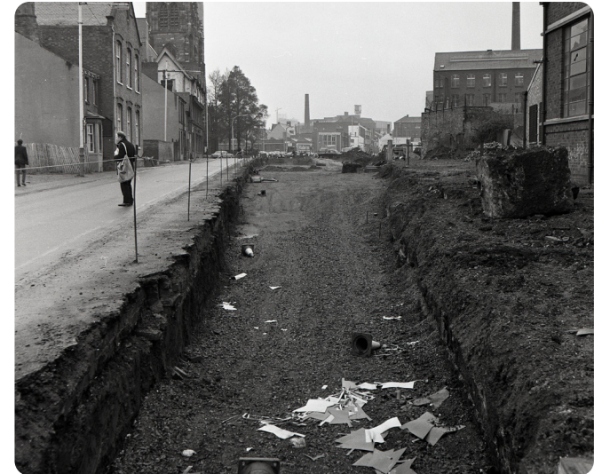
Figure 12: Construction of St. Margaret's Way, 1969
