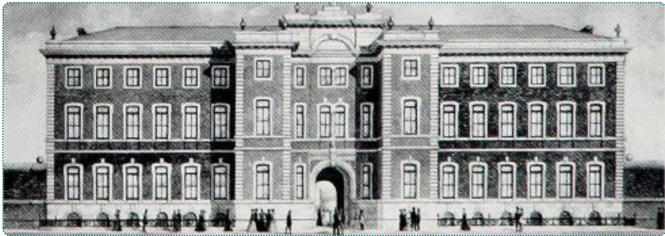
Figure 23: The 1865 Factory Building Designed by William Jackson
