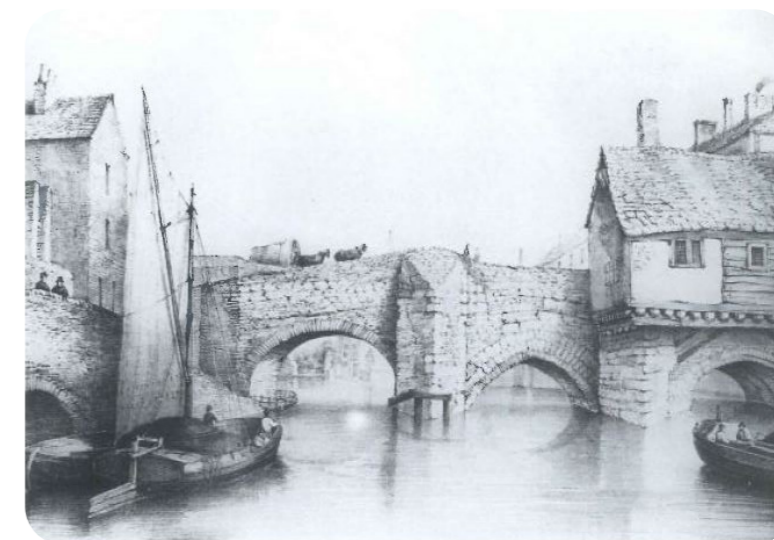
Figure 137. The old West Bridge from around 1841 (Malcolm Elliot: Leicester - A Pictorial History)
