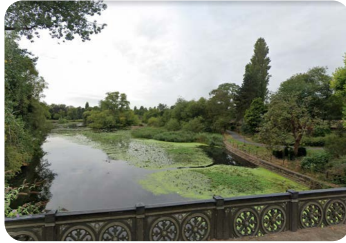
Figure 461. APVP6. Note: Abbey Park Road Bridge Closed for repairs. (Image taken from Google)
