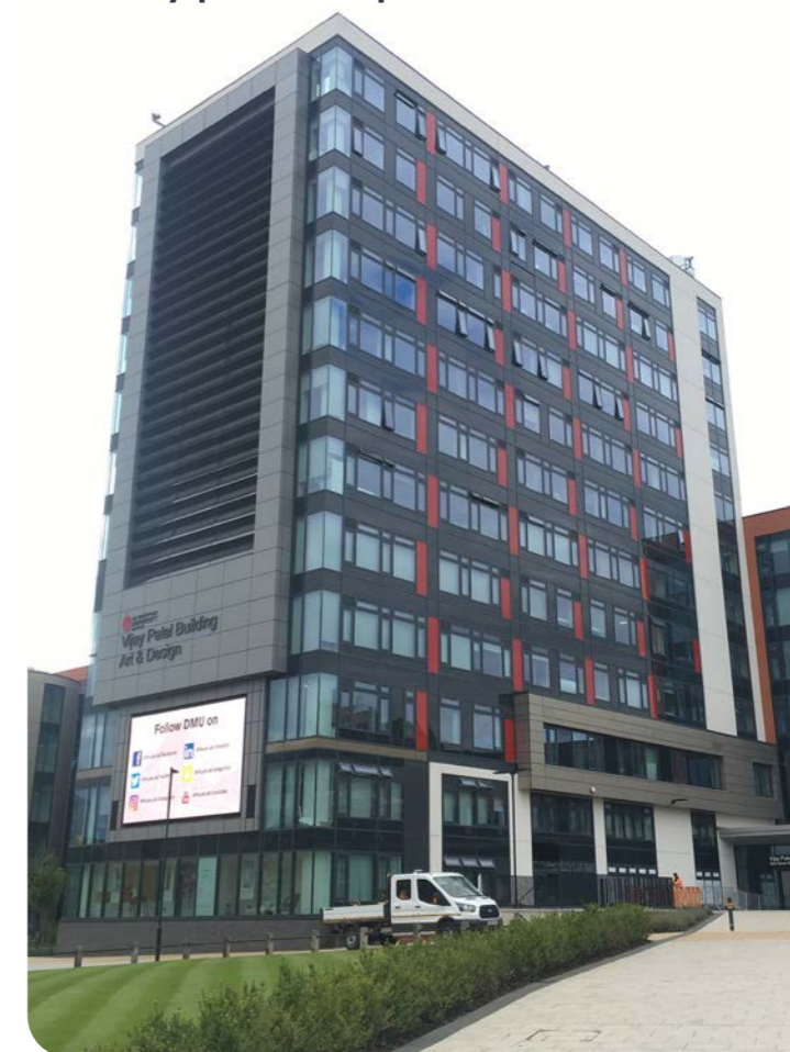
Figure 20. The Vijay Patel Building, De Montfort University, part of a comprehensive scheme.
