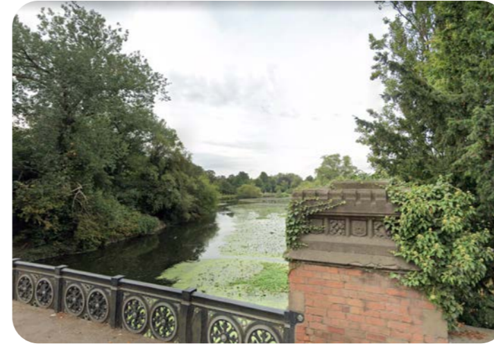
Figure 462. AP VP7. Note: Abbey Park Road Bridge Closed for repairs. (Image taken from Google)
