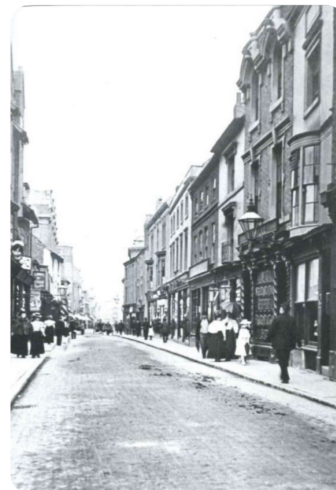
Figure 159. High Street in the early 1900s with the Clock Tower in the distance taken before it was widened (Ben Beazley: Leicester Then and Now)
