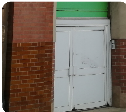
Glazed Brick Plinths
